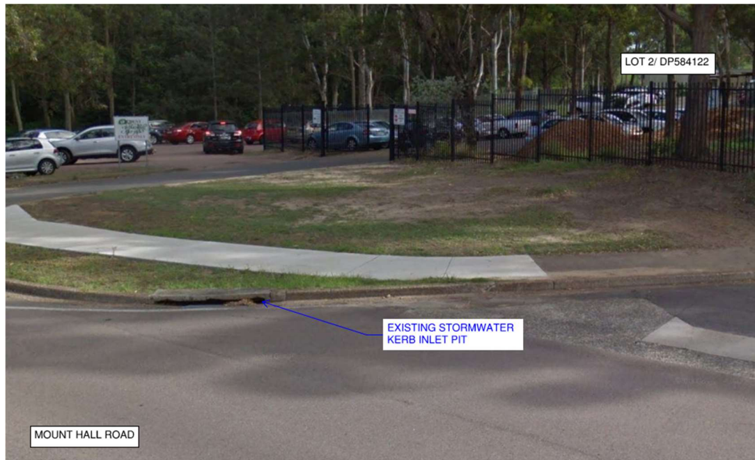
Figure 3: Existing Stormwater Infrastructure (Google Maps, 2018)
